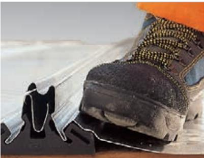
Stand on top of the profile to ensure the panels are properly connected.
