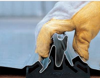
Place the overlapping edge of the next panel into the clip by repeating step 1.
