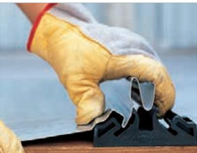
Once the panel is completely secured to the first run of clips, insert the second run of clips to the free side of the panel (gutter side for Riverclack® 500 and Riverclack® 550, overlapped side for Riverclack® Grip 600).
