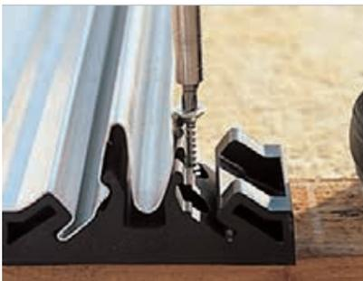
Secure the clips to the supporting element using the appropriate fixings.
