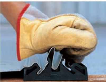
2. Push down carefully on the top until the panel locks into the clip (you should feel a "click"). The panels themselves determine the correct location of the clips.
